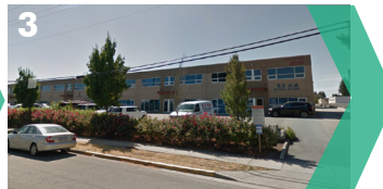
3 Sale and disposition of existing facility at 2633 Simpson Road, Richmond.
